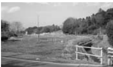
▲大関調整池下流付近
